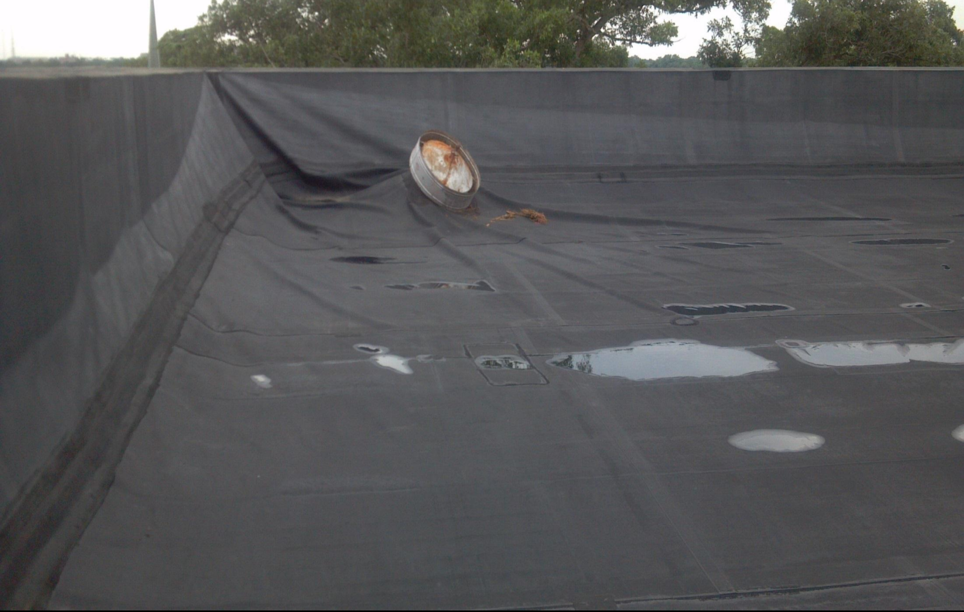
DHHS – Dix McBryde – EPDM roofing membrane failure.
