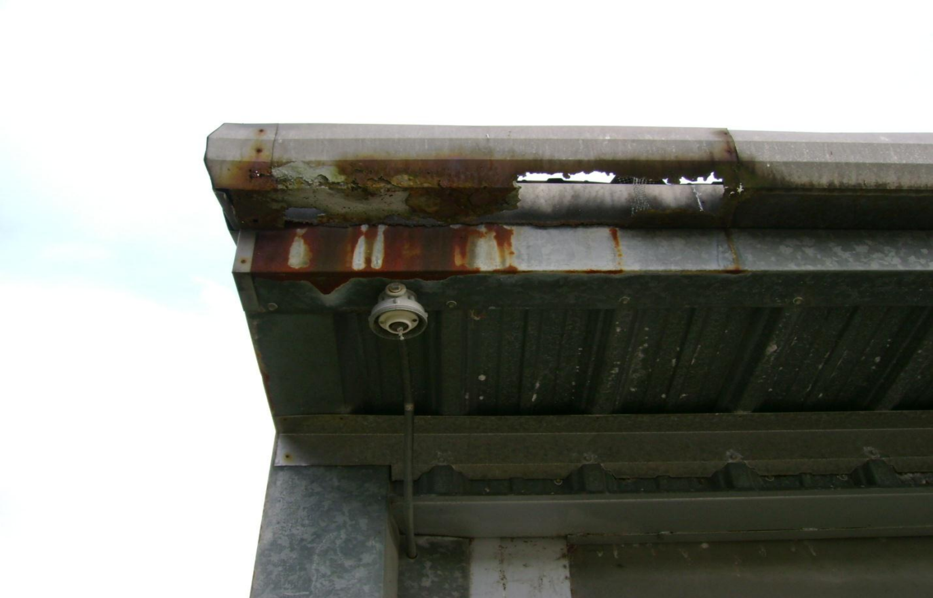
DHHS – Caswell Center – Gutter rusted through which causes roof water to pond against the building.
