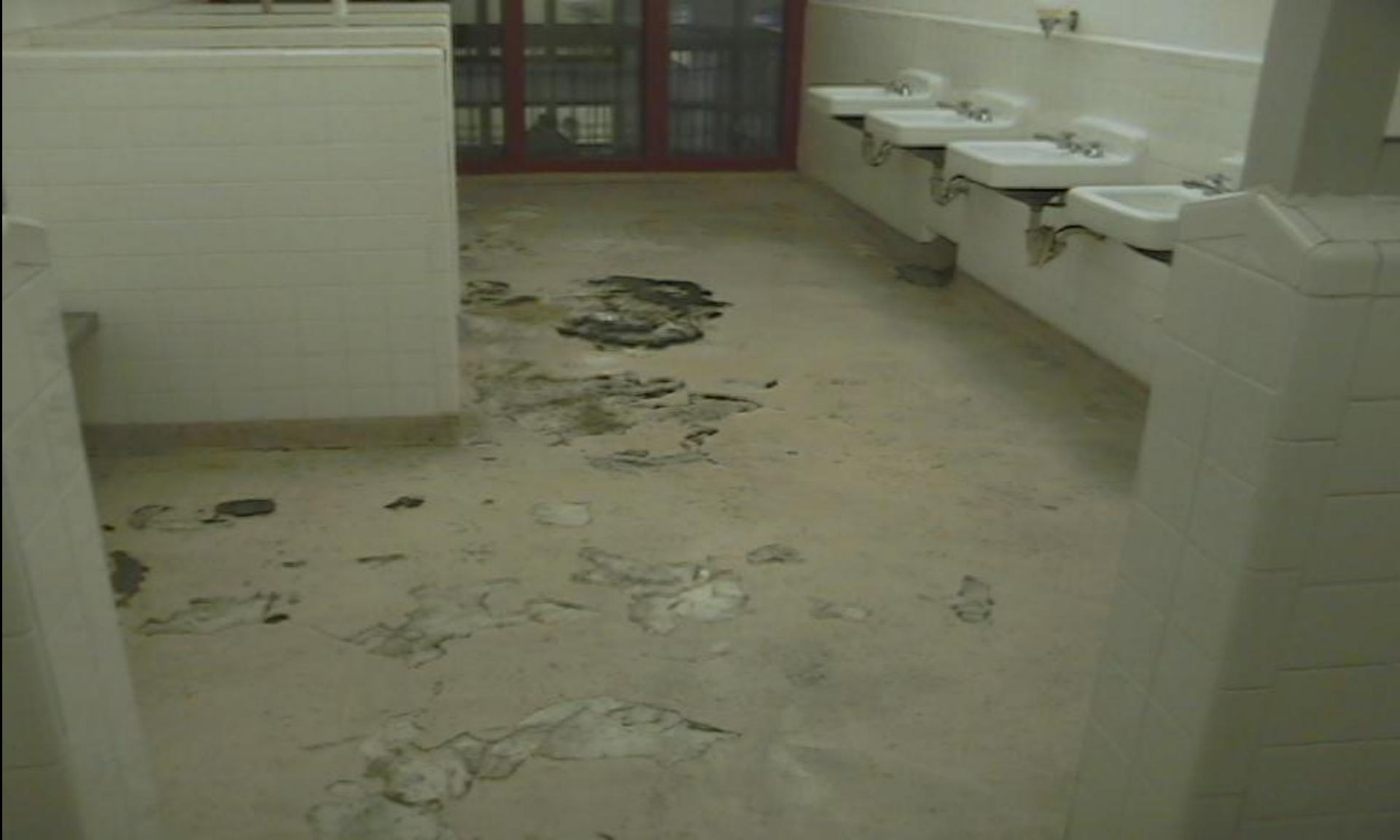
DPS – Hyde Correctional – Bathroom flooring worn and needs replacement.
