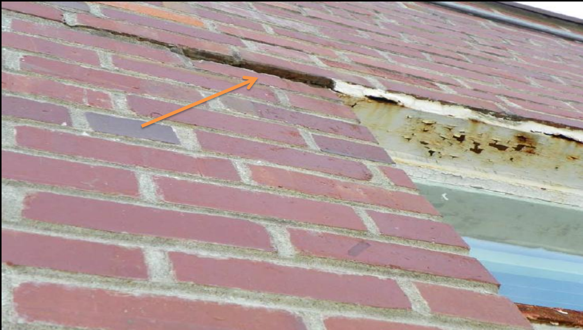
DPS – Dobbs Youth Development Center – Rusting lintels above windows causing structural problems. Typical across the state.
