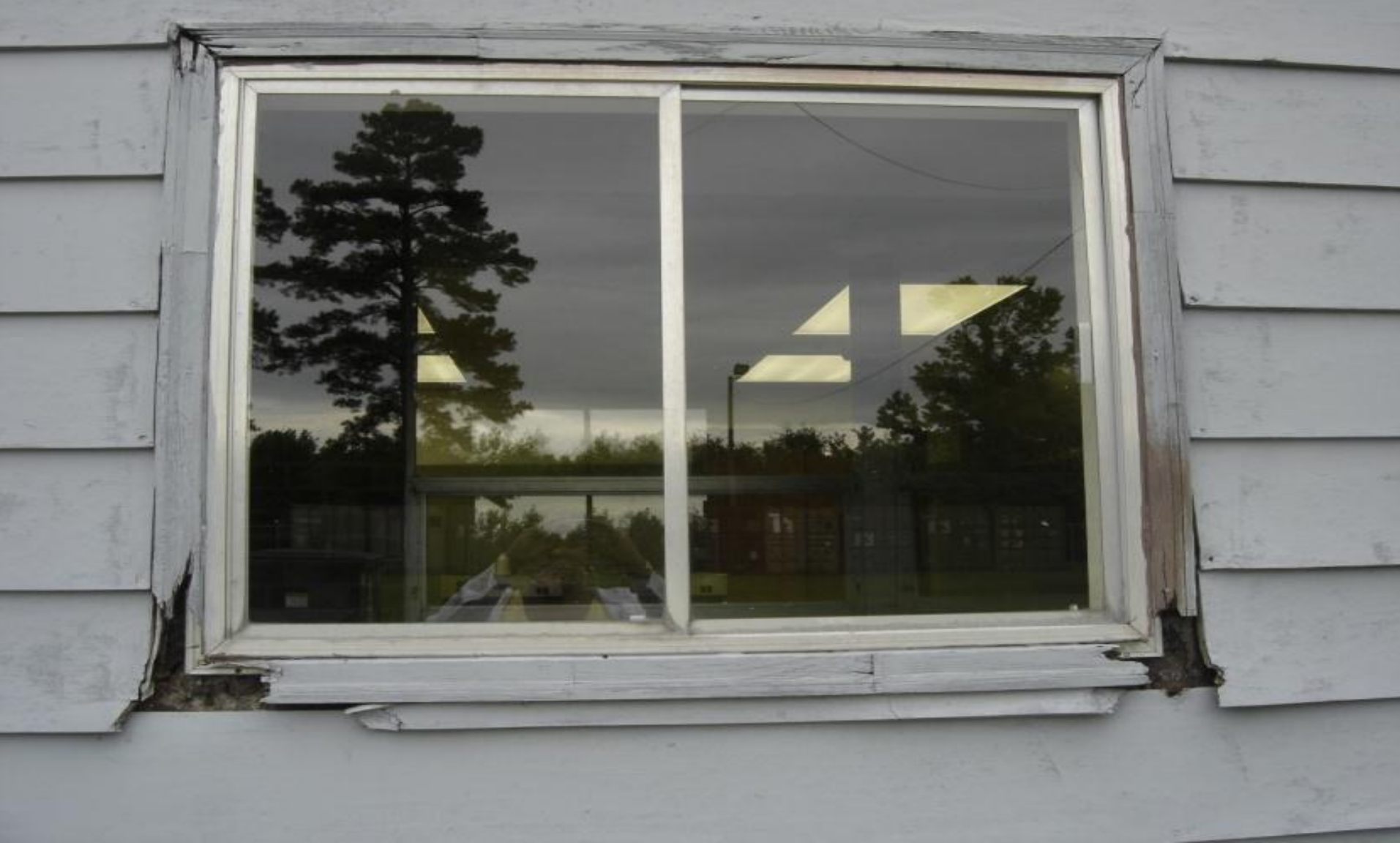
DPS – NCNG – Beulaville – Water infiltration due to rotting siding and window trim.
