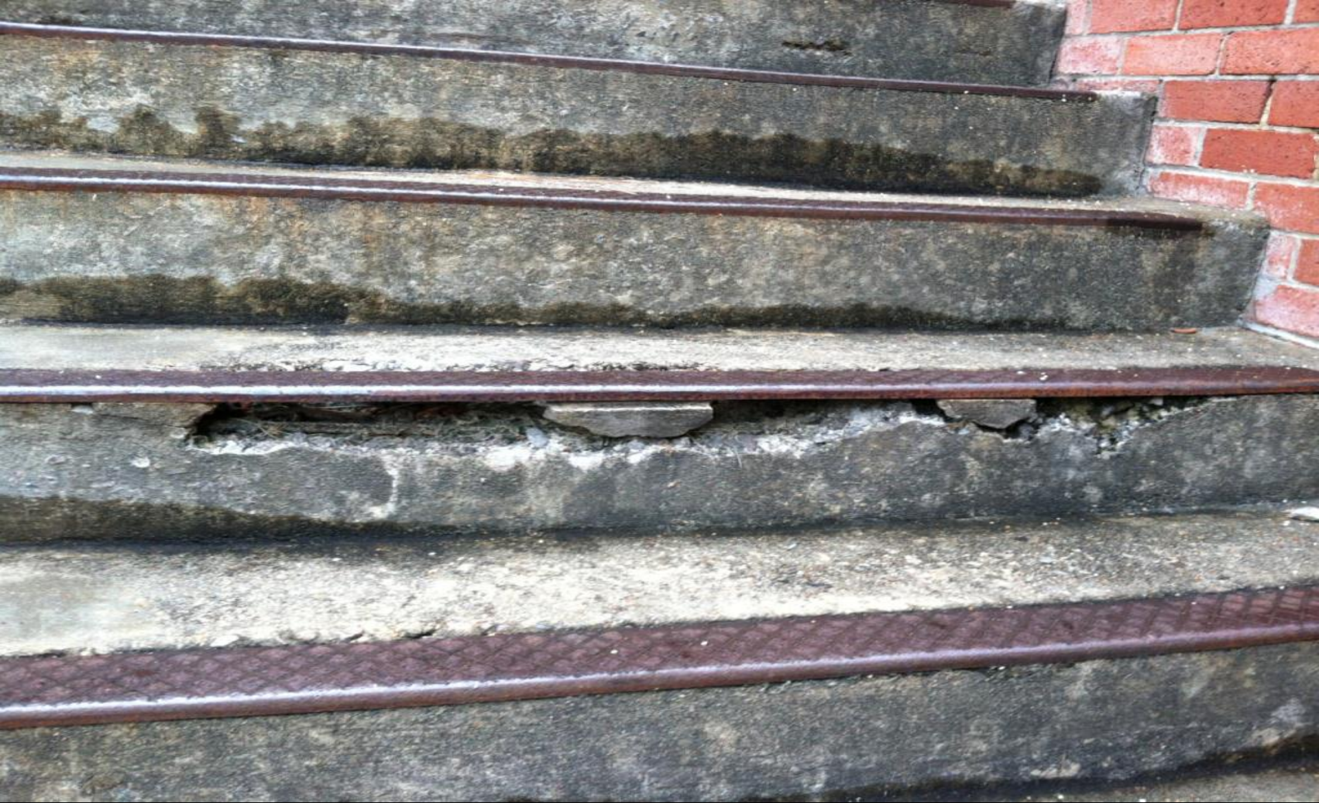
NCCU – Turner School of Law – Rusted stair nosing and deteriorated concrete steps. Safety hazard.
