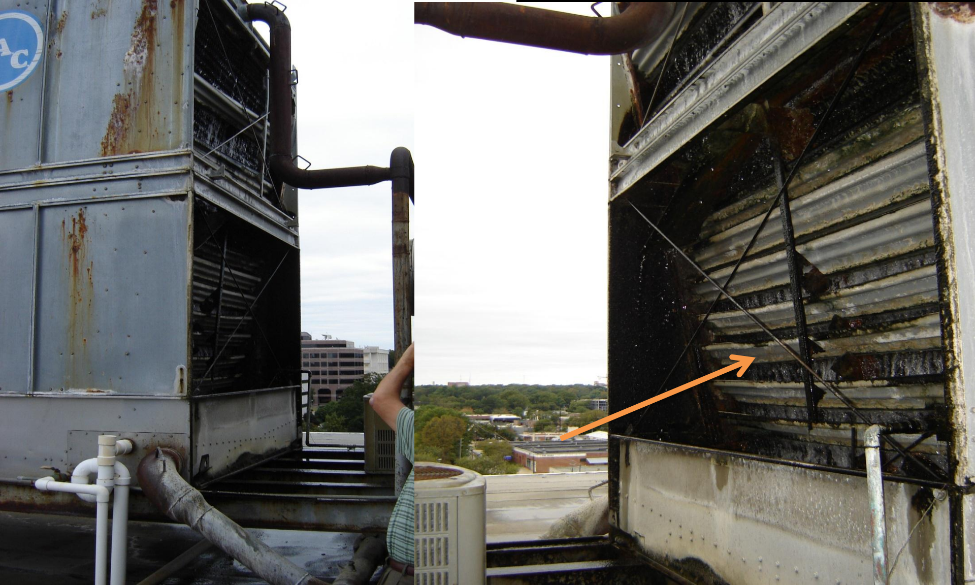
DOA – Shore Bldg – Cooling tower past is useful life. Rusted and broken supports.
