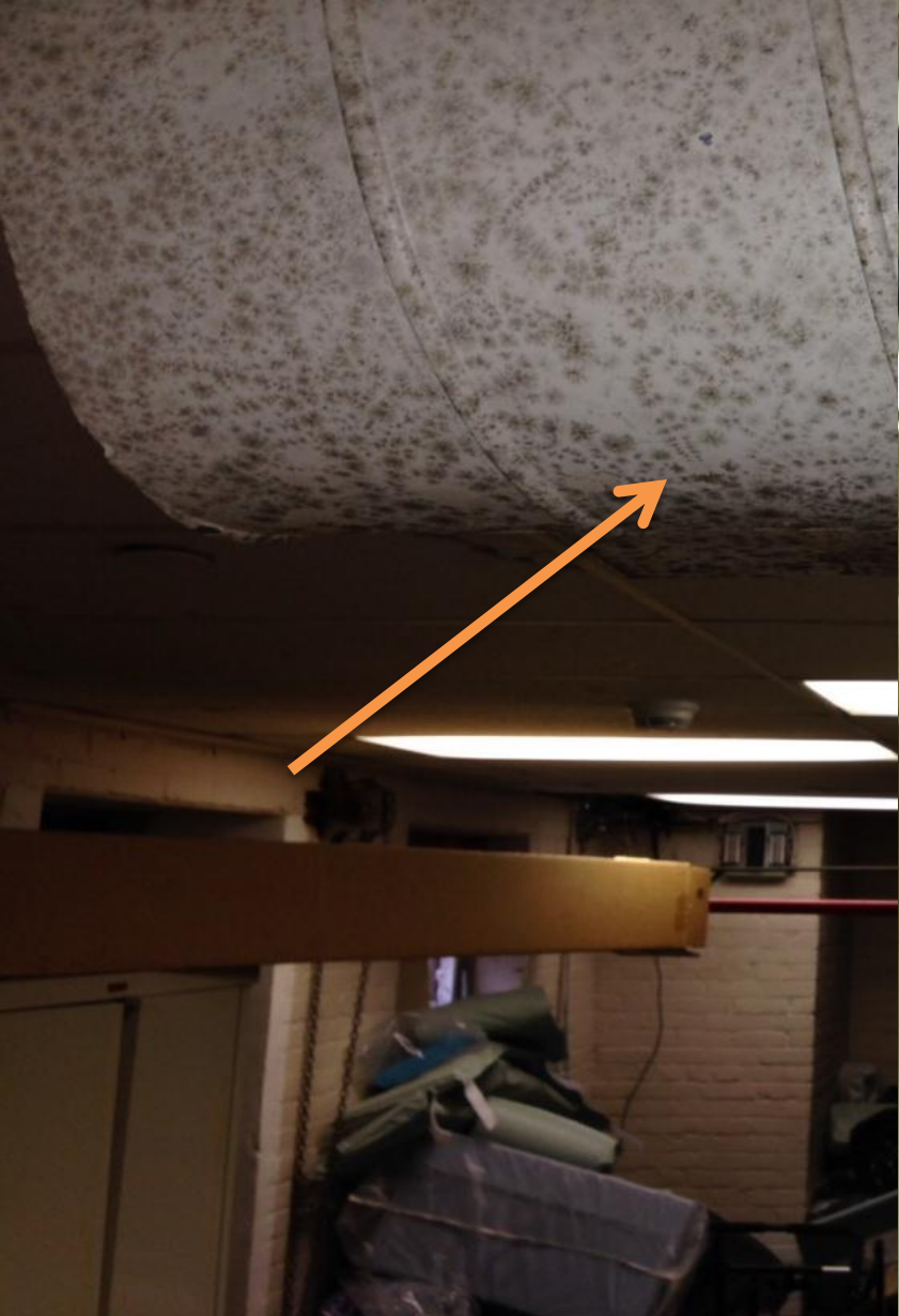
DHHS – Black Mtn. Neuro-Medical Treatment – Moldy ducts.
