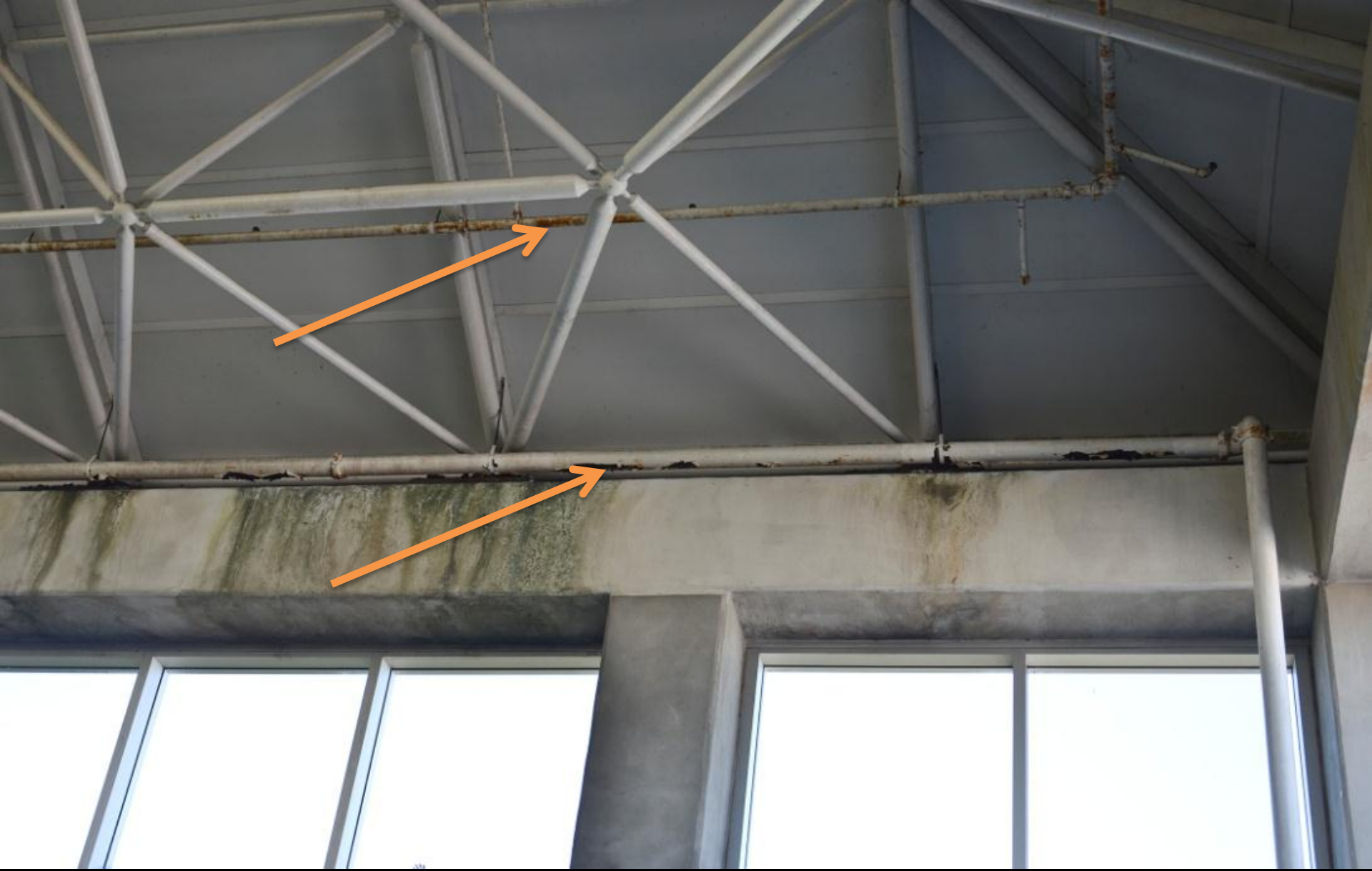
DENR - Fort Fisher Aquarium – Fire sprinkler pipes in the conservatory are corroding as a result of exposure to the salt air.
