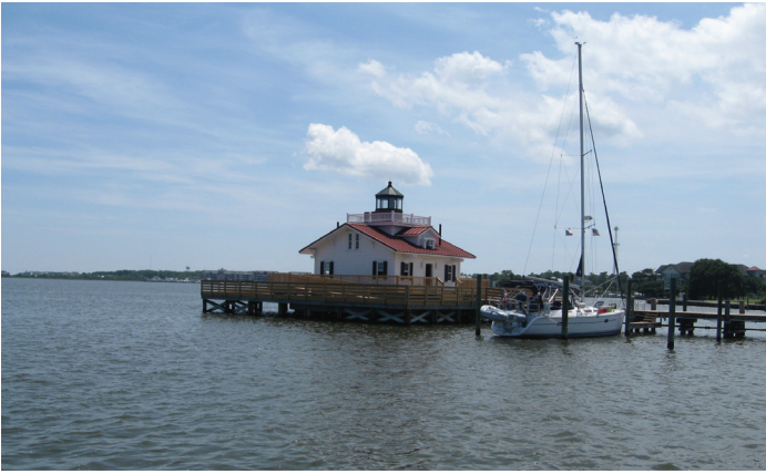
Roanoke Marshes Lighthouse, Town of Manteo
