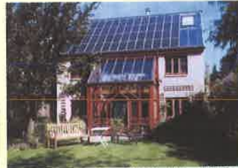
Figure 3.24 In this solar house in Oxford, UK, a 1 MWp grid-linked array of monocrystalline PV modules forms an integral part of the roof, alongside solar water heating panels. The PV array supplies the house's annual electricity requirements, plus a small surplus used to provide some of the power for a small electric car
