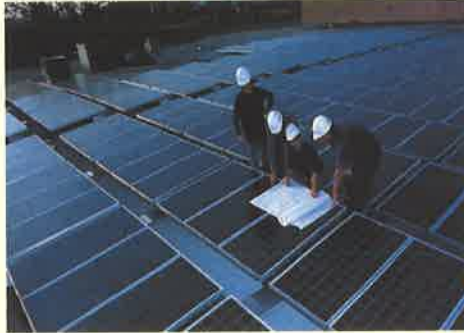
Figure 3.24 In this solar house in Oxford, UK, a 1 MWp grid-linked array of monocrystalline PV modules forms an integral part of the roof, alongside solar water heating panels. The PV array supplies the house's annual electricity requirements, plus a small surplus used to provide some of the power for a small electric car
