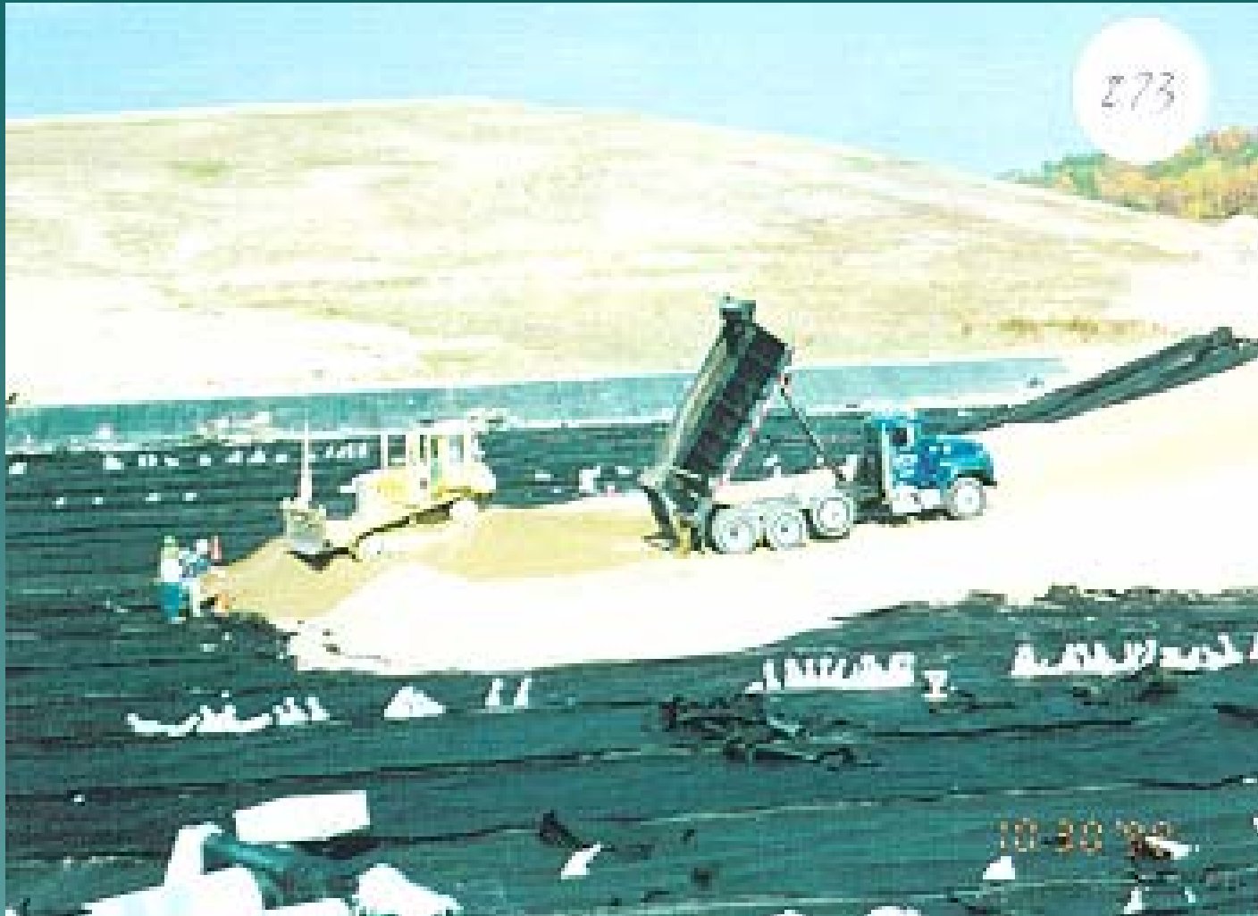
Leachate Collection - Granular Drainage and Protective Layer
