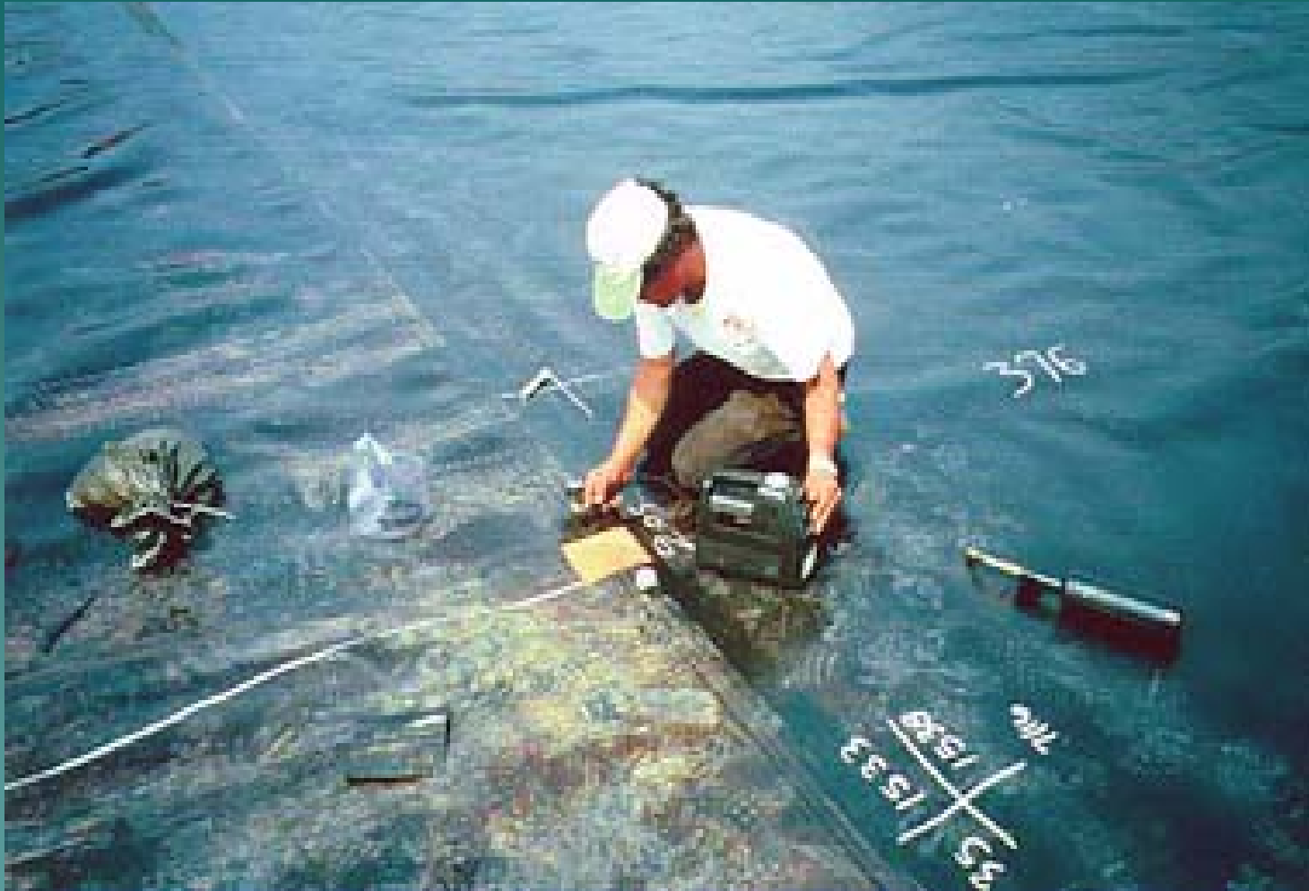
Seam Testing - Air Pressure
