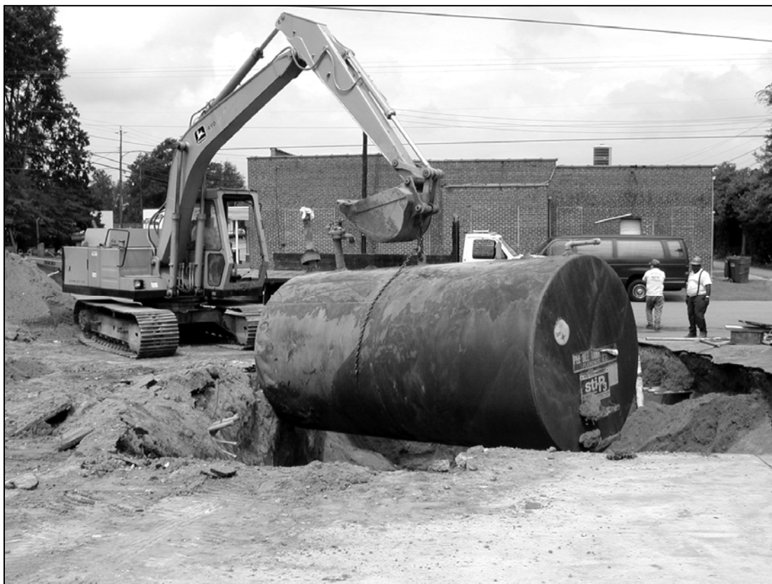
UST Release Incident-Tank Removal
