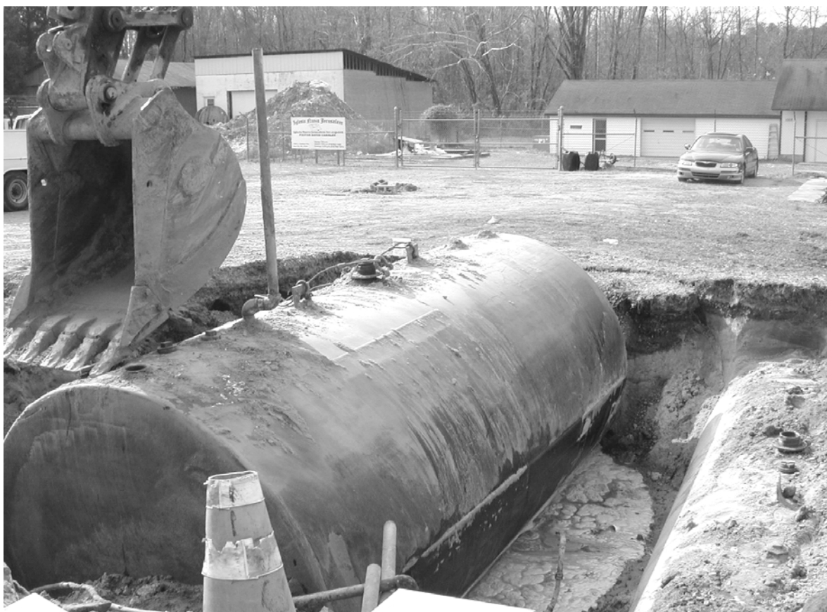
UST Release Incident-Kerosene Free Product in Basin
