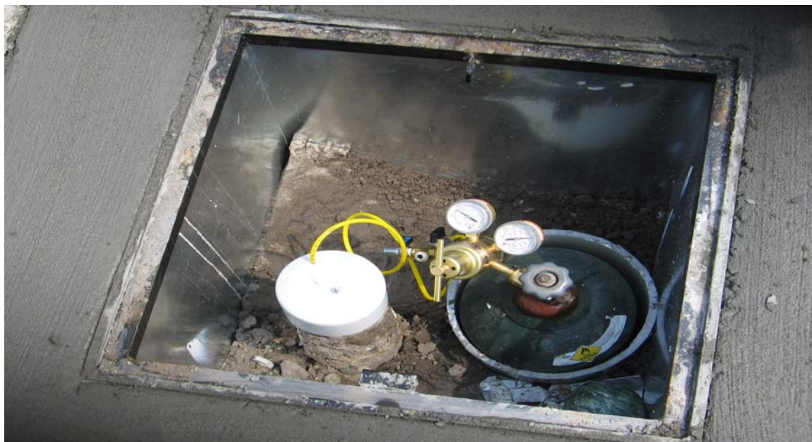
(A completed iSOC well vault with oxygen cylinder. Courtesy of Pyramid Environmental & Engineering, PC.)
