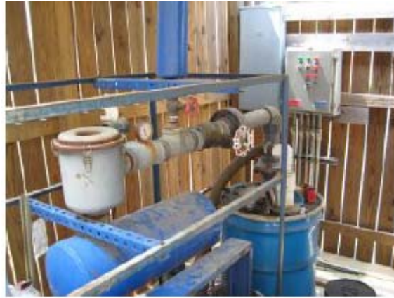
Photo 6: SVE knock out tank and control panel
