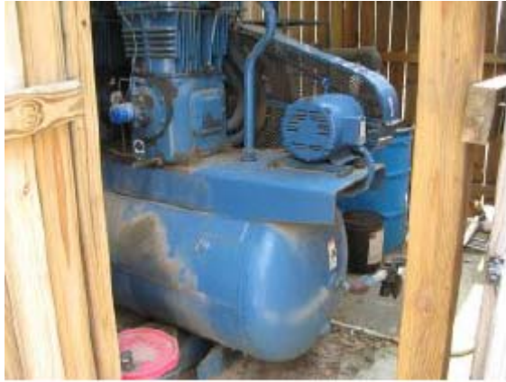
Photo 5: Air sparge compressor unit
