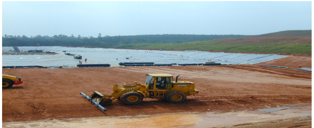
Landfill liner installation
