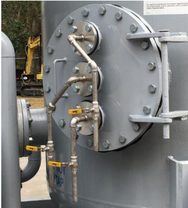
Figure 4. 25%, 50% and 75% Bed Depth Sampling Ports
