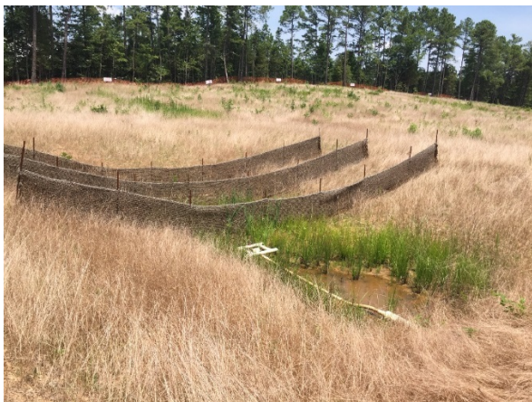
Figure 7 - Good Vegetative Stabilization
