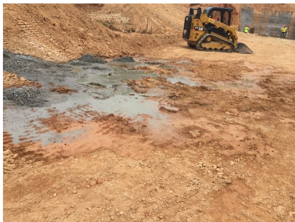
Figure 1 - Unmanaged Concrete Washout Area
