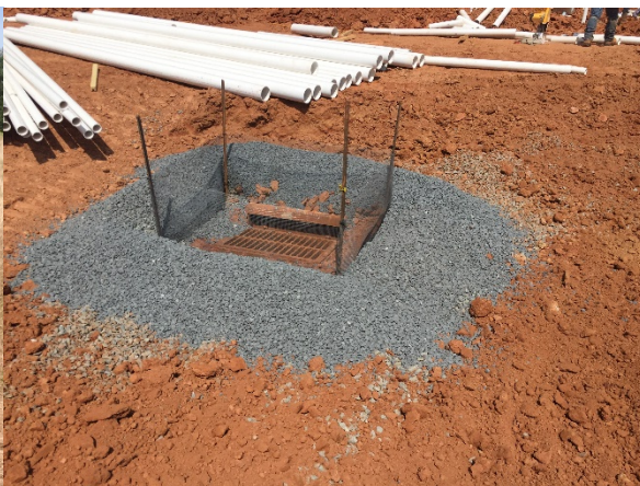
Figure 8 - Good Inlet Protection
