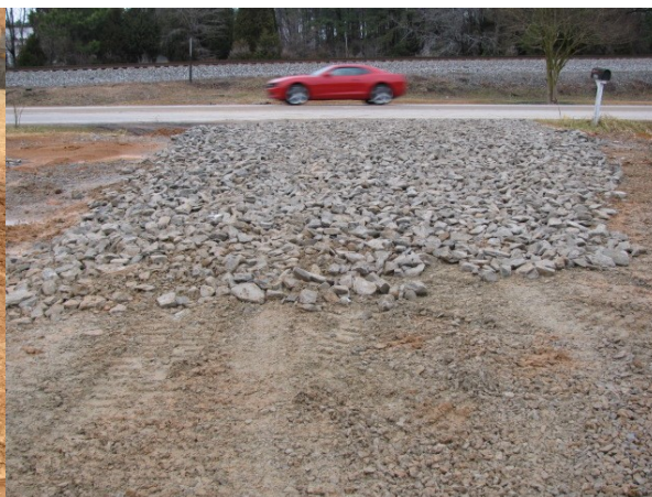
Figure 2 - Good Construction Entrance
