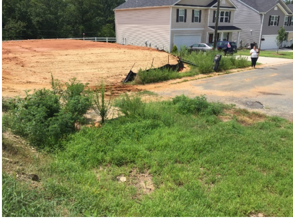
Figure 3 - Poor Practice - No Construction Entrance
