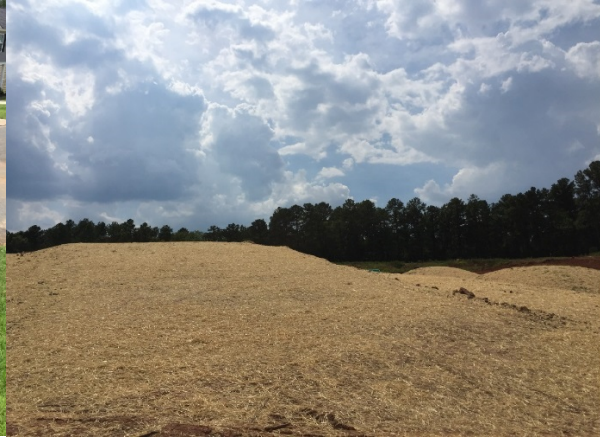
Figure 4 - Example of Good Application of Ground Cover
