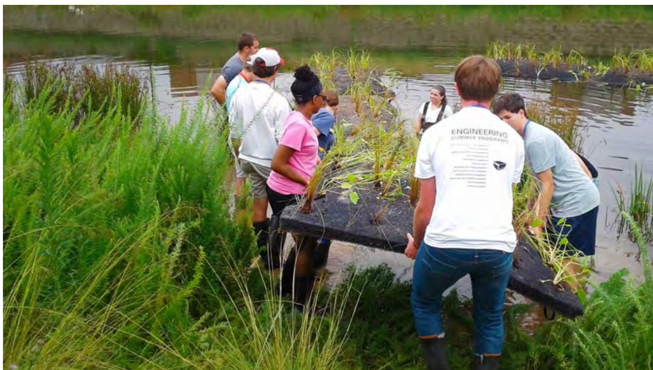
N.C. State students installing a Floating Treatment Wetland.
