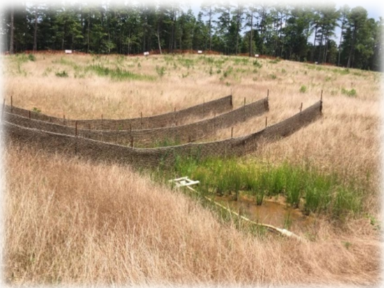
Figure 12 - Good Vegetative Stabilization
