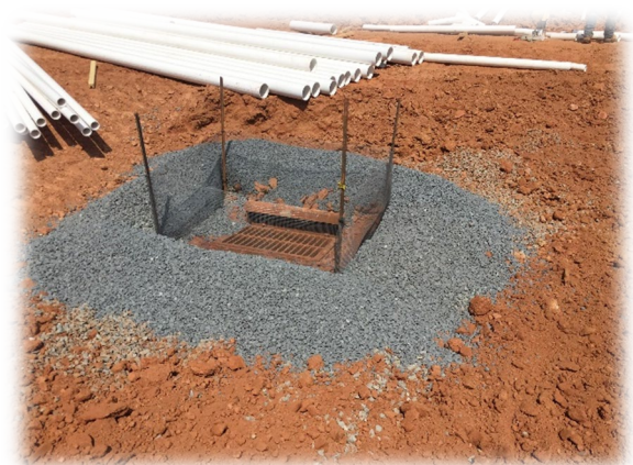
Figure 13 - Good Inlet Protection
