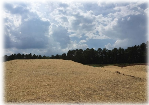
Figure 9 - Good Application of Ground Cover
