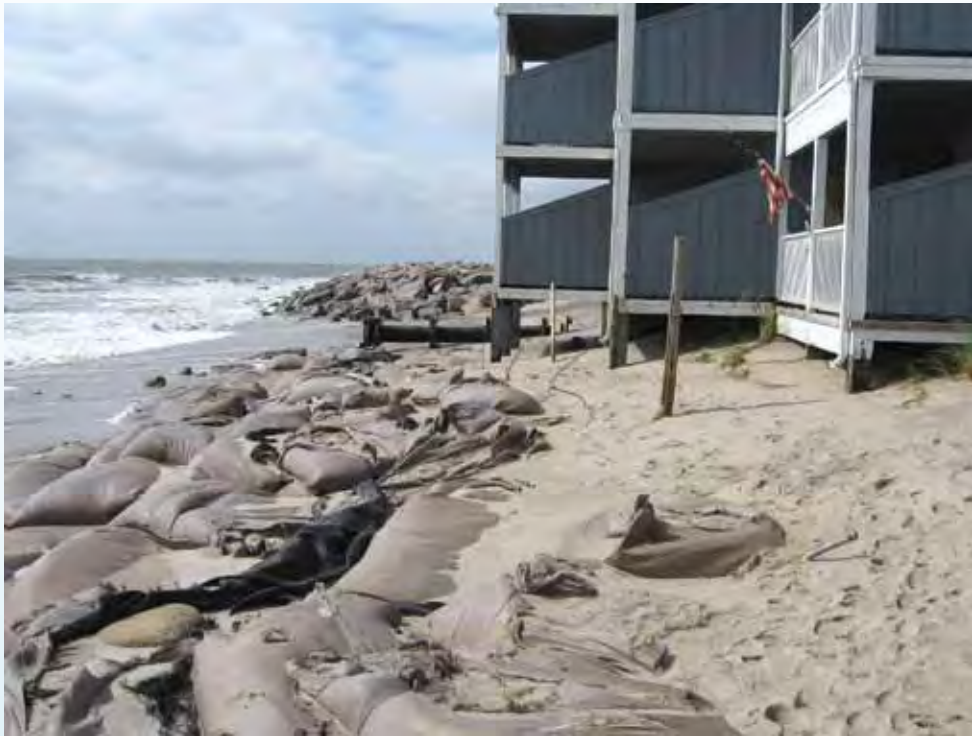
Using sandbags for temporary erosion control requires a CAMA permit. N.C. Division of Coastal Management.
