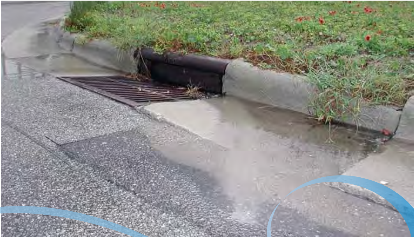
Runoff that flows down the storm drain goes directly to a nearby body of water, along with any pollutants it may be carrying. N.C. Division of Water Quality.
