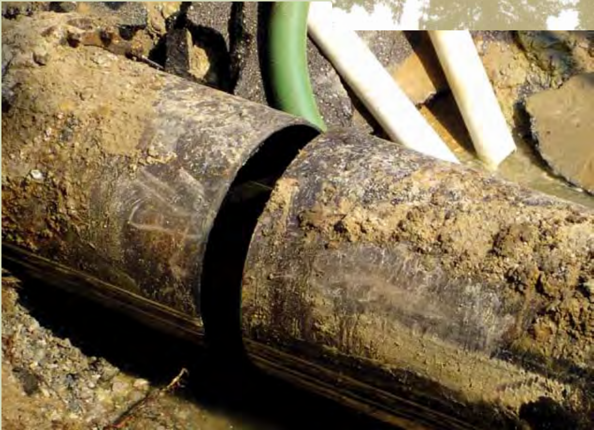
Pipe separation at Hewlett’s Creek. N.C. Division of Water Quality.
