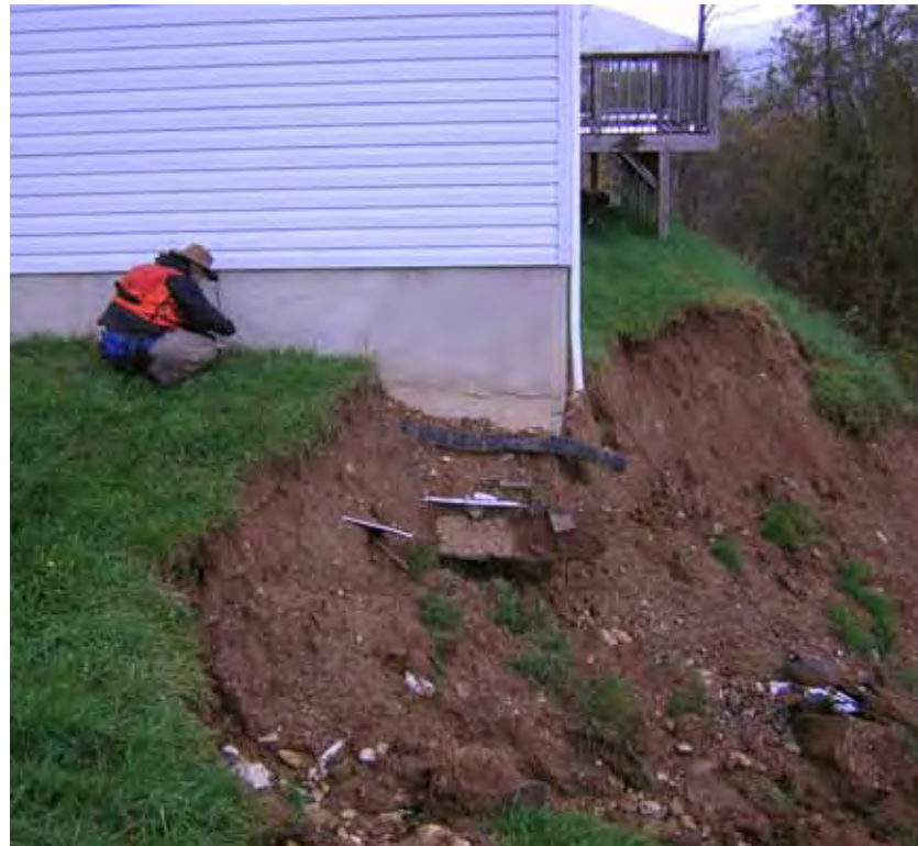
Rebecca Latham of the N.C. Geological Survey takes notes about the landslide that occurred in the White Laurel subdivision of Watauga County. Notice that the landslide shown began under the corner of the house, cracking the foundation. N.C. Division of Land Resources.
