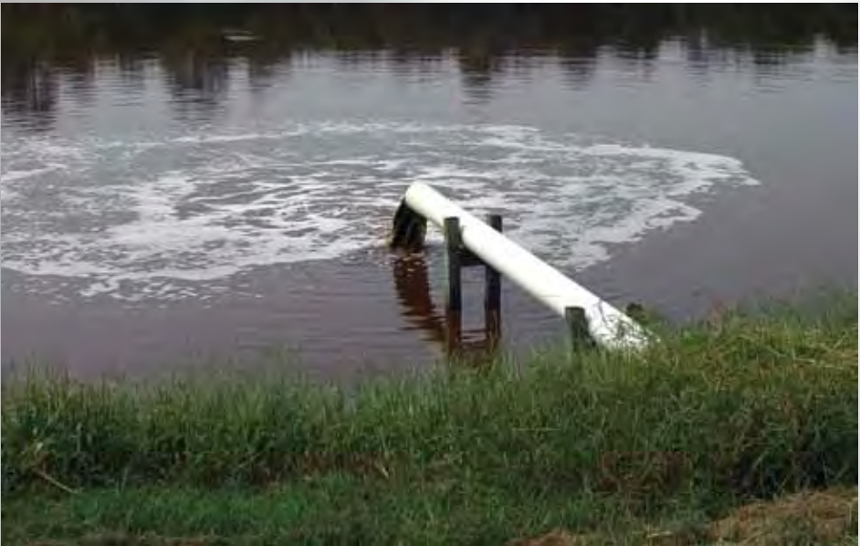
A flush pipe runs from the swine barn into the lagoon. N.C. Division of Pollution Prevention and Environmental Assistance.
