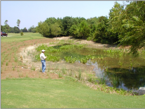
Stormwater wetland, New Hanover County
