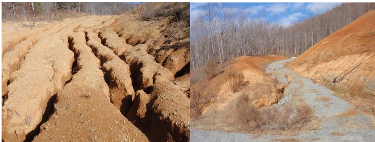
Examples of abandoned construction sites with eroding roadways and slopes causing offsite sedimentation.
