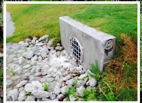
Outfall at Level Spreader, Pine Knoll Shores East End Drainage Project (CS370717-01)
