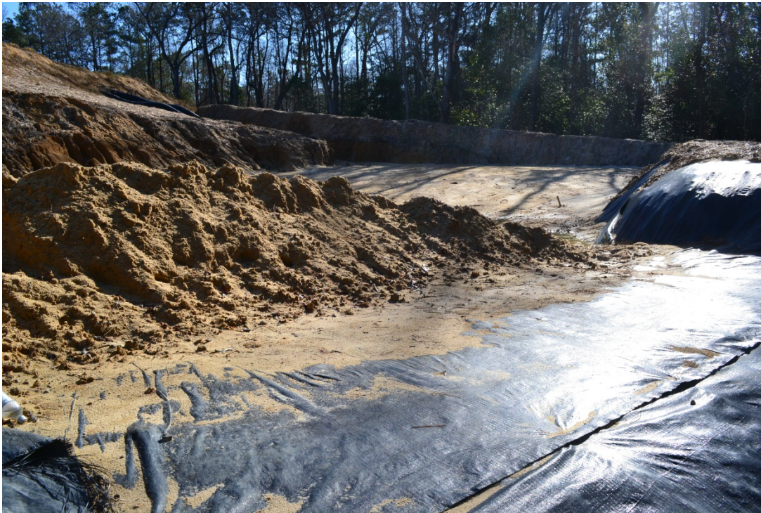
Unmaintained Sedimentation Basin filled to the brim with sediment.
