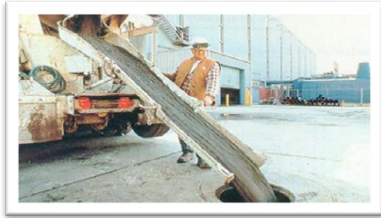
Flowable fill application (Headwaters Resources, Inc.)
