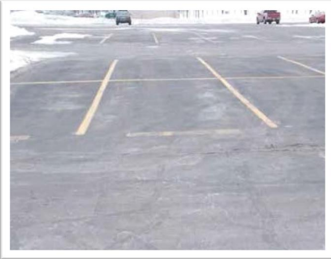
Photo of parking lot eight years after repairs using Class C fly ash and reclaimed asphalt (ACAA).
