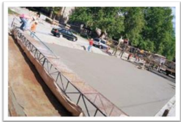
Fly ash concrete finishing (www.fhwa.dot.gov)
