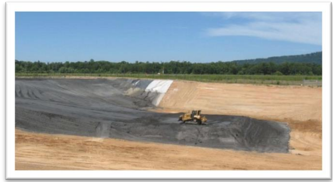
A liner is laid out at the Asheville Regional Airport as part of a structural fill that has used approximately four million tons of coal ash in the airport expansion project. (NC Department of Environment and Natural Resources)
