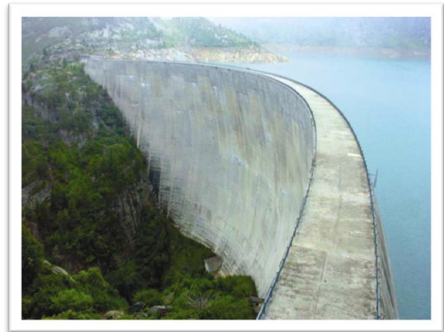
At 318 feet tall, the Olivenhain Dam is the largest roller-compacted concrete dam of its kind in North America.
