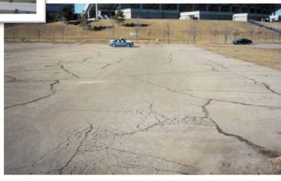
Deteriorating asphalt pavement at Jack Trice Stadium.
