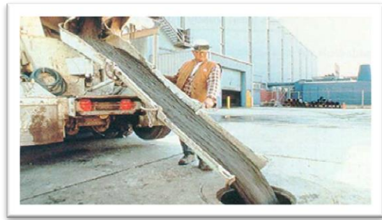
Flowable fill application (Headwaters Resources, Inc.)
