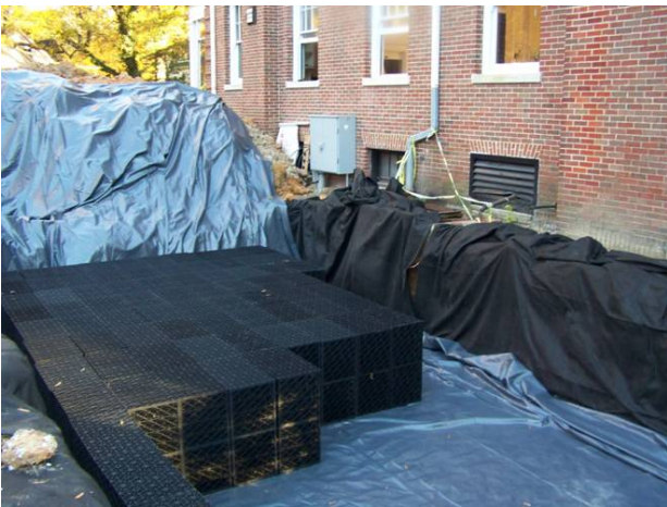
Installation of cisterns – Durham
