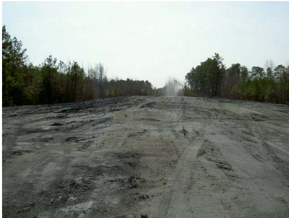
CCP Structural Fill under construction in Halifax County
