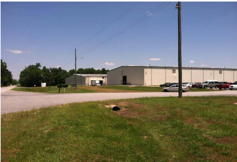
EB Grain Warehouses constructed on CCP Structural Fill on Hwy 301 north of Rocky Mount.
