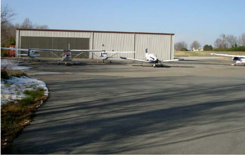
Structural Fill used for construction of airport hangar at Lake Norman Airport.
