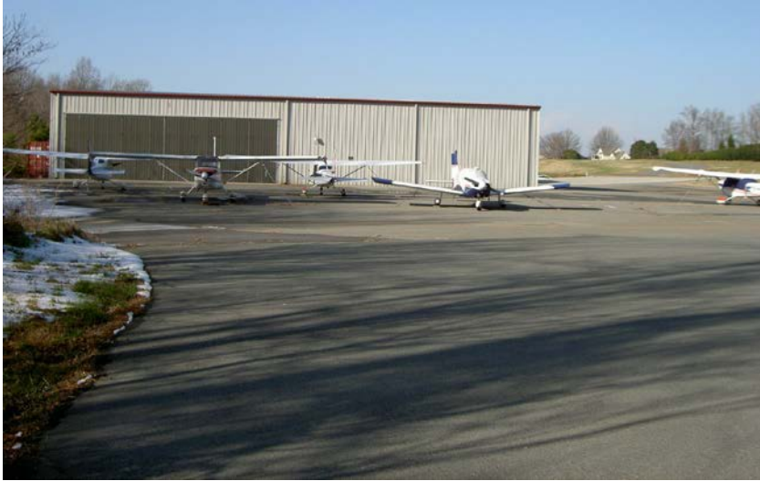
Structural Fill used for construction of airport hangar at Lake Norman Airport.
