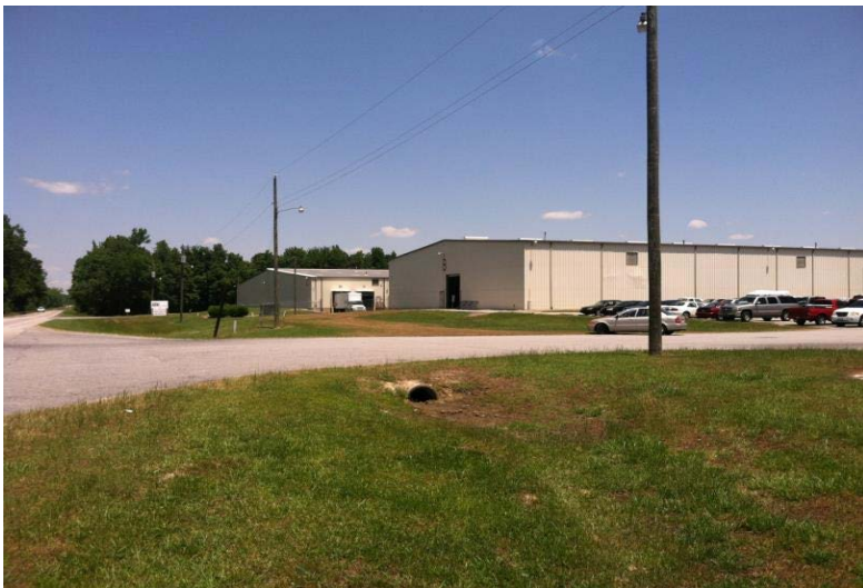
EB Grain Warehouses constructed on CCP Structural Fill on Hwy 301 north of Rocky Mount.
