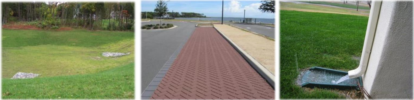
Figure 16: Excellent Options for Bacteria Removal & Water Quality in General: Infiltration Systems, Permeable Pavement and Disconnected Impervious Surfaces (NCSU)
