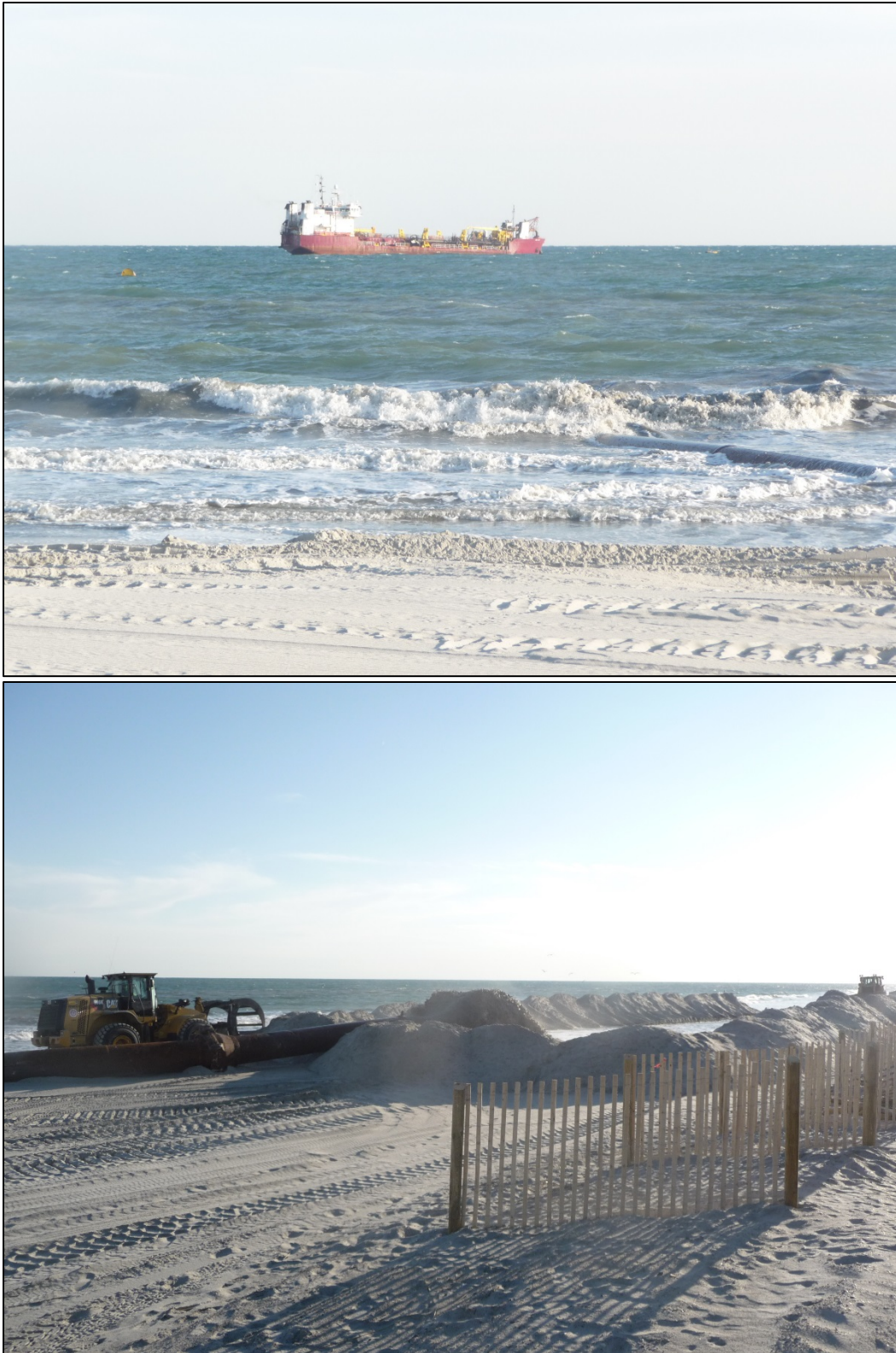
Figure III-63. Hopper Dredge Operation (Bogue Banks)
