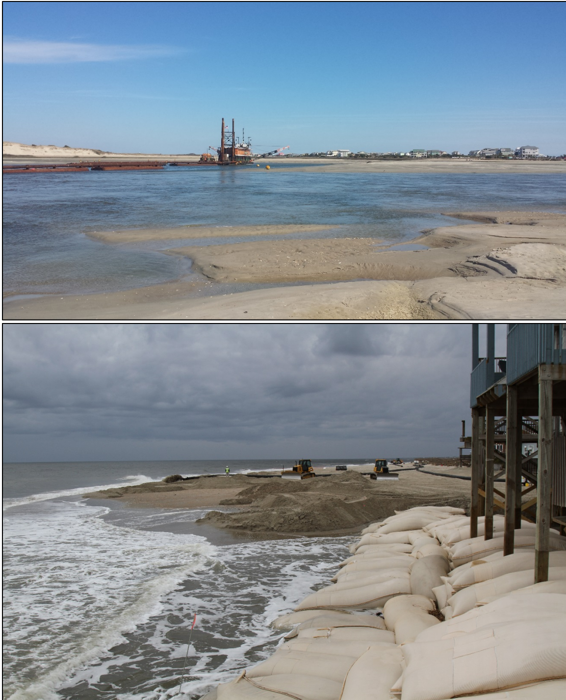
Figure III-62. Cutter Suction Dredge Operation (Oak Island)
