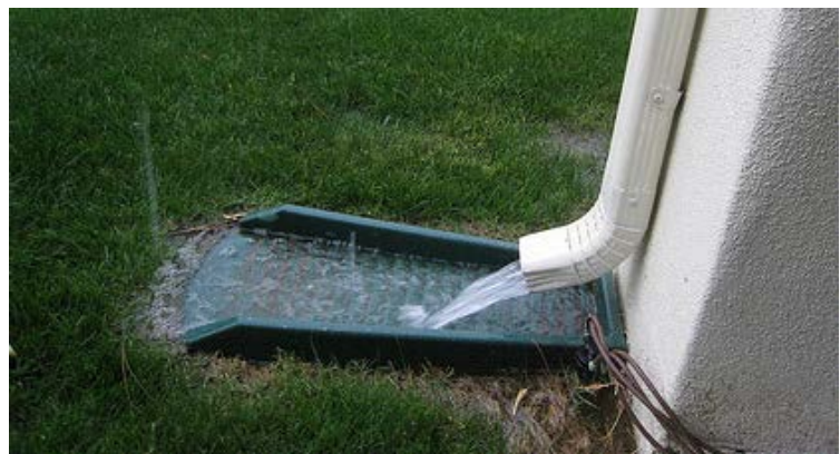
Figure 3: DIS – A Simple and Cost-Effective SCM
