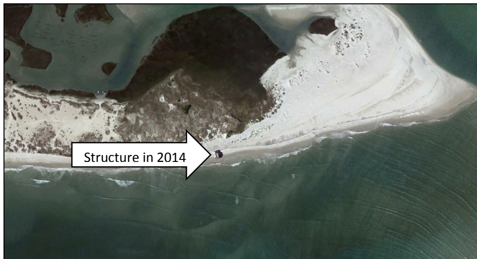
Figure 8. In 2014, the same structure identified in Figure 7 sat on the ocean's edge at low tide until finally being destroyed by a storm in 2015 (Photo source: Google Earth 2014).
