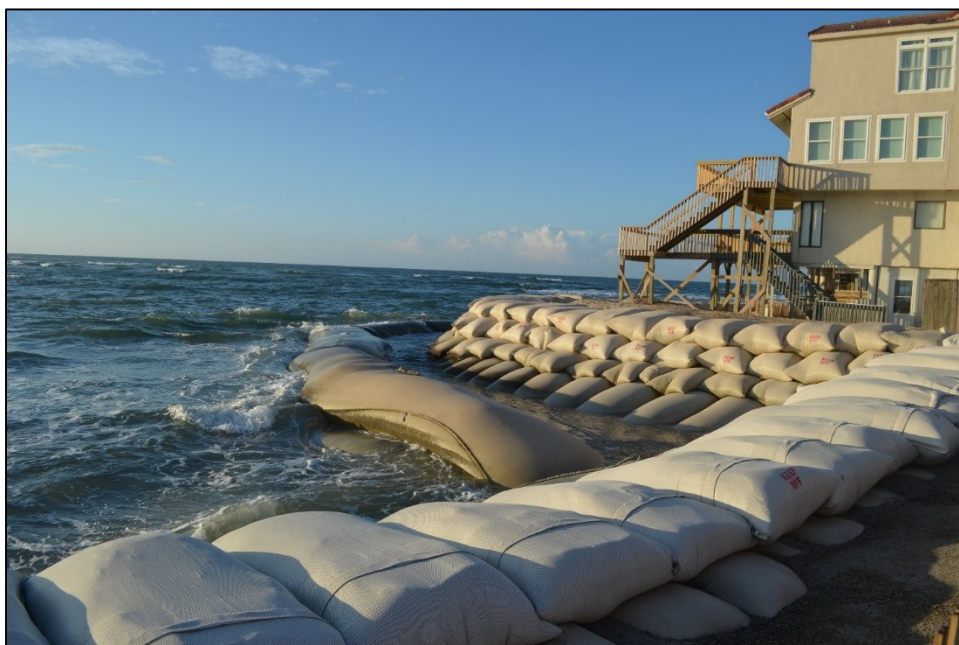
Figure 22. Sandbag structures at North Carolina's North Topsail Beach have been successful in providing short-term home protection from erosion at the expense of losing a sandy beach. Photo: NCDCEM, 2015
