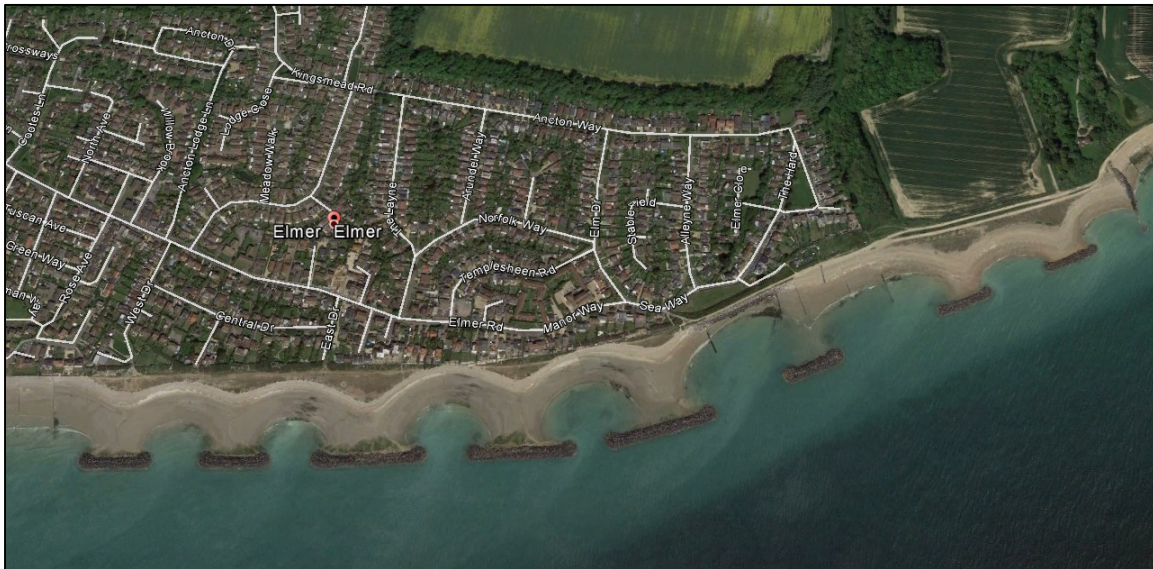
Figure 17. Breakwaters installed at Elmer, UK. Although erosion appears to be reduced, these structures do interfere with sediment transport causing a “scallop effect” on the beach as sediment fills in behind each breakwater.
