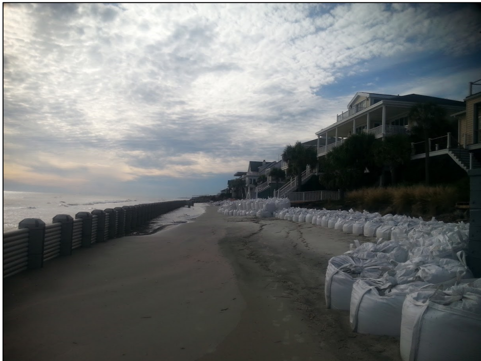
Figure 16. Experimental structure at Isle of Palms, S.C., installed in front of sandbags. Photo: NCDCM, 2015
