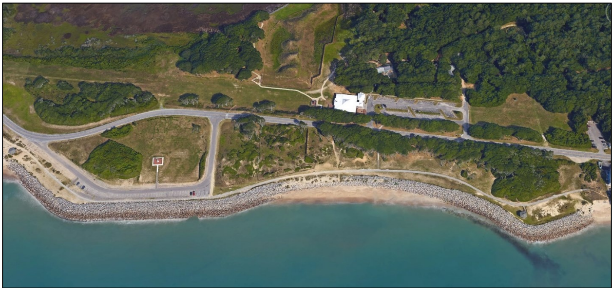
Figure 13. Fort Fisher State Park, N.C. rock revetment. Photo: NCDWM
