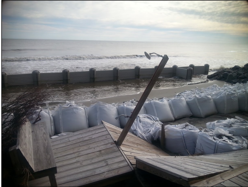
Figure 15. Experimental structure at Isle of Palms, S.C. Photo: NCDCM, 2015
