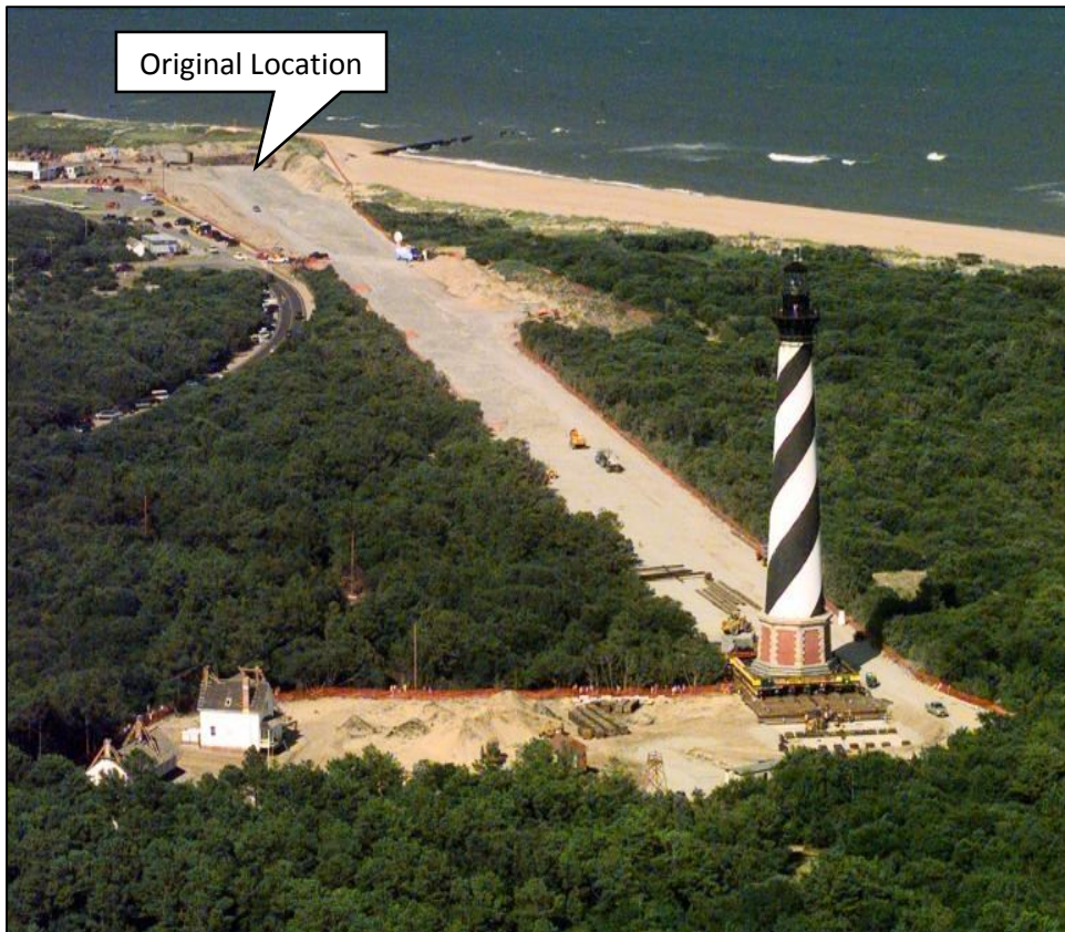
Figure 2. Cape Hatteras Lighthouse after being moved (1999). Photo: National Park Service
