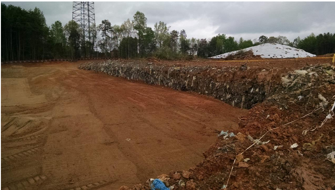
Mooresville, N.C. site where a pre-regulatory landfill was discovered by a contractor installing a detention pond
