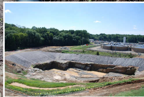
Construction at the Muddy Creek WWTP in Winston-Salem (CS370399-08)
