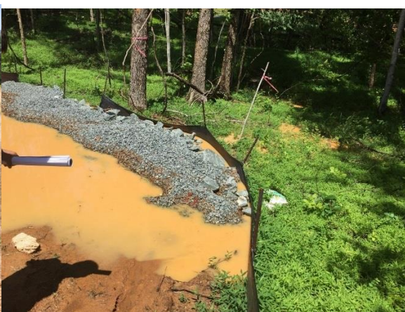
Figure 8 - Silt Fence Outlet in Wrong Location
