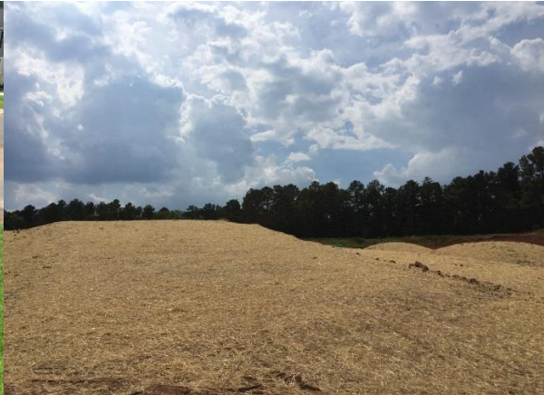
Figure 4 - Example of Good Application of Ground Cover
