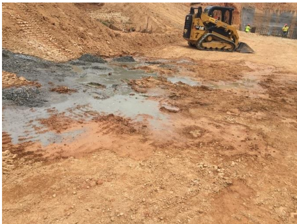
Figure 1 - Unmanaged Concrete Washout Area
