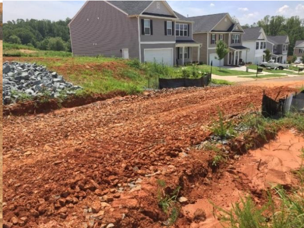
Figure 2 - Construction Entrance needs maintenance
