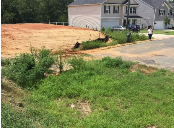
Figure 3 - Poor Practice - No Construction Entrance
