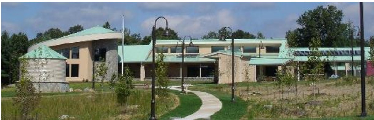
Figure 2: Rainwater harvesting system at the Wilkes County Rest Area (on the left)
