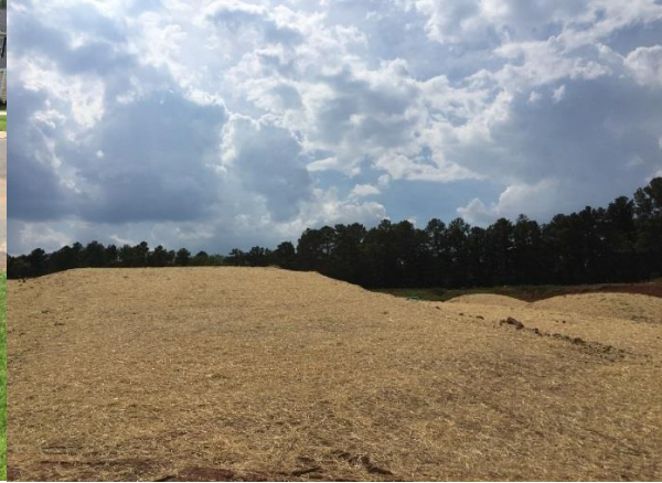
Figure 4 - Example of Good Application of Ground Cover
