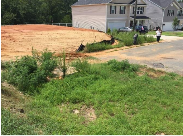
Figure 3 - Poor Practice - No Construction Entrance
