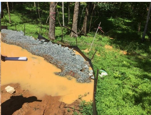
Figure 8 - Silt Fence Outlet in Wrong Location
