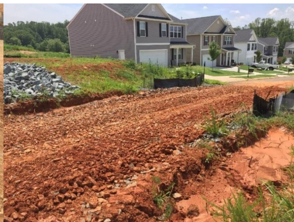
Figure 2 - Construction Entrance needs maintenance
