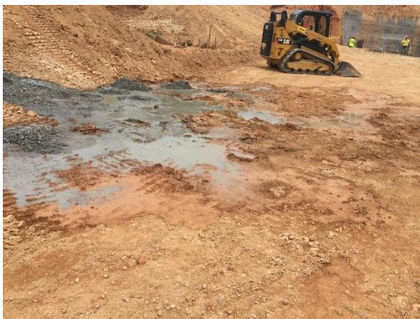
Figure 1 - Unmanaged Concrete Washout Area
