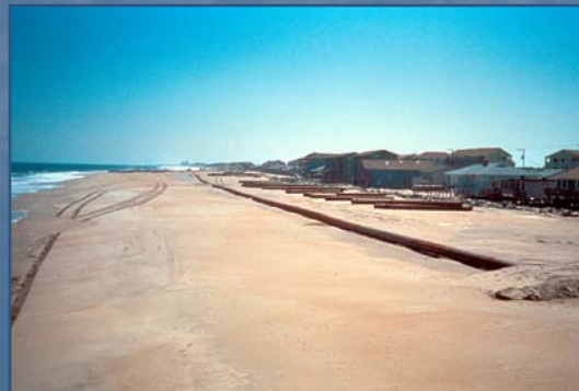
Fed, State, Local mitigation
