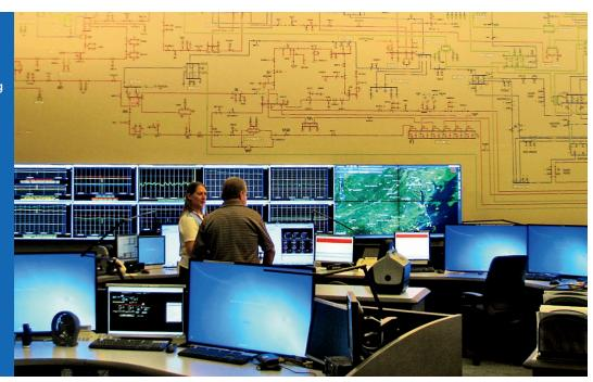
IMPORTANT FACILITY — The SOC is the brains of the system and performs real-time monitoring of the transmission grid to maintain reliability. Operators communicate with the regional transmission organization (PJM), Dominion's Regional Operations Centers, and other interconnected distribution and transmission companies.
