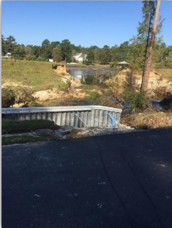
Embankment Breach
