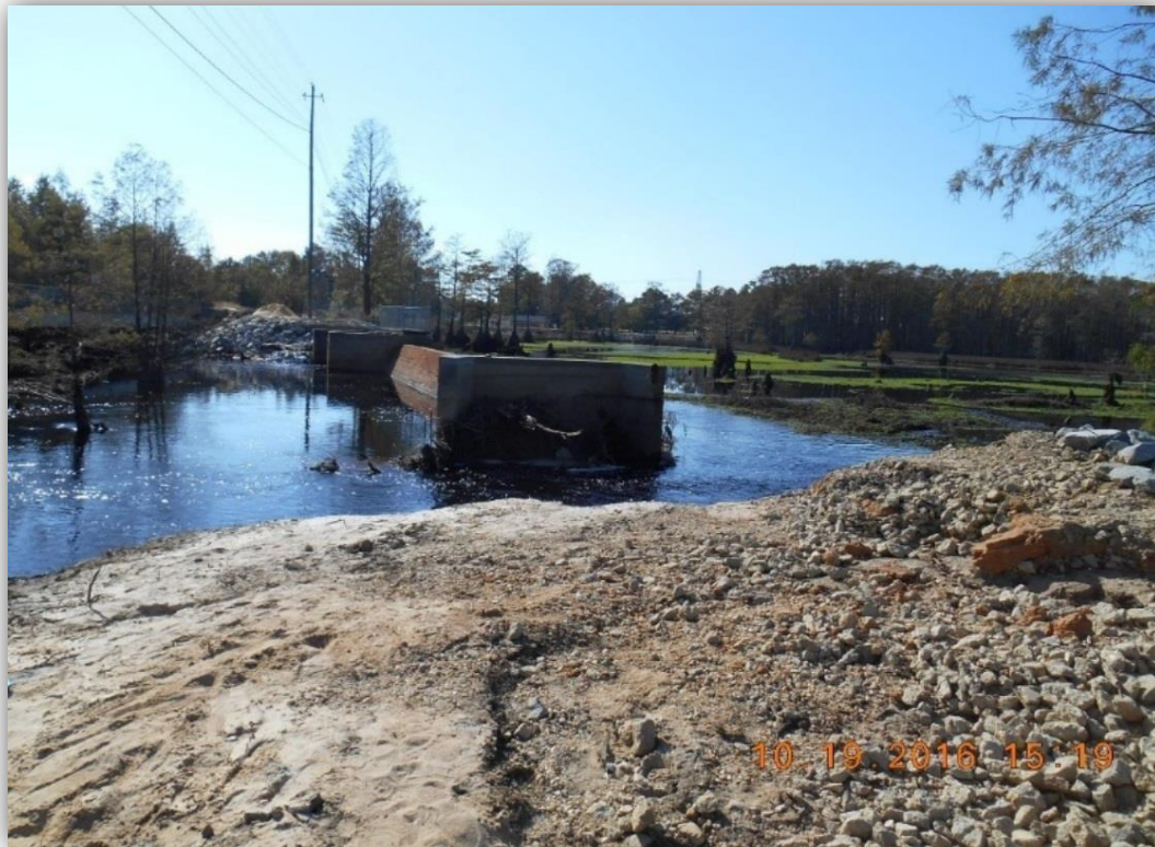
Spillway Abutment Wall Breach
