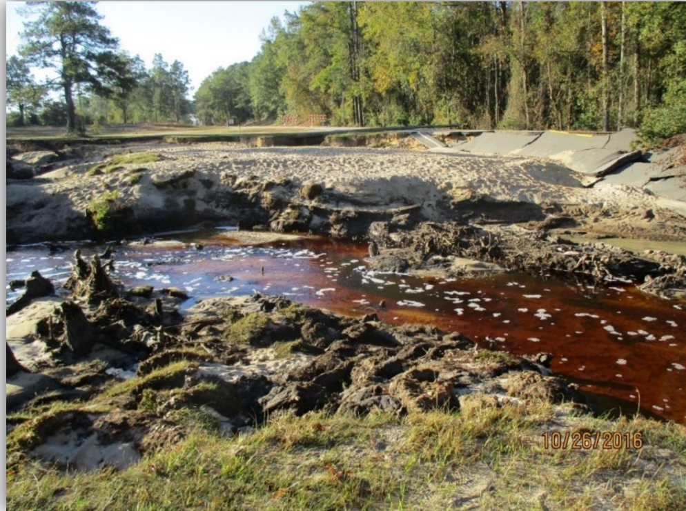
Dam Embankment Breach / Highway 53 Taken Out
