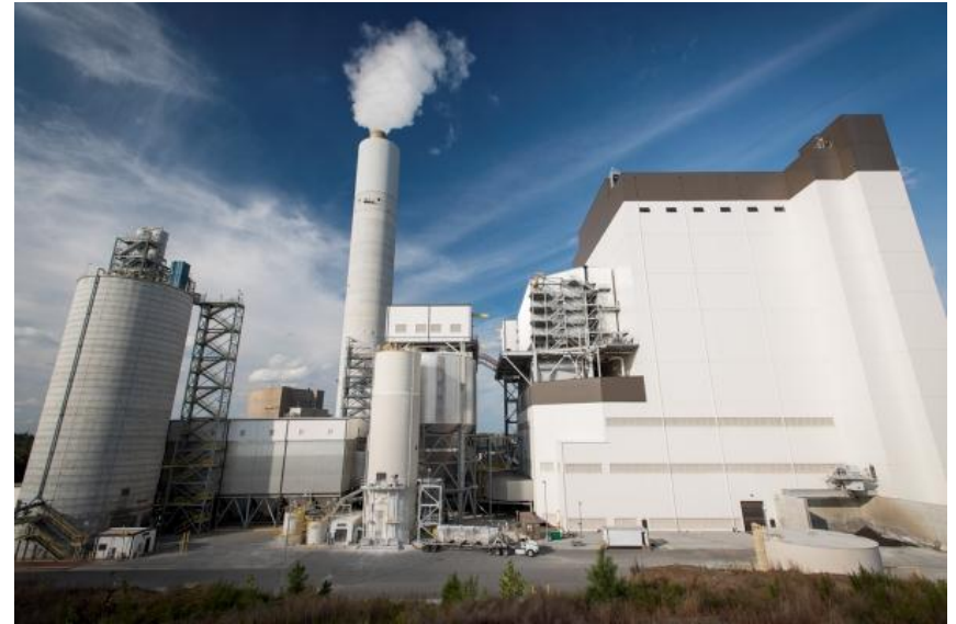
Cliffside Unit 6 is among the newest and cleanest coal plants in the nation
