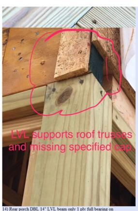
14) Rear porch DBL 14" LVL beam only 1 ply full bearing on post: ONE PLY STILL 1 3/4" SHORT.
