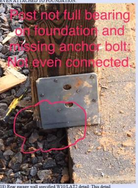
18) Rear garage wall specified W10/LAT2 detail: This detail is for a load bearing wall with uplift. The rear wall is a non-bearing wall with no uplift: Plans/design needs to match construction: STILL NEED PLANS AND DETAILS THAT MATCH CONSTRUCTION.
