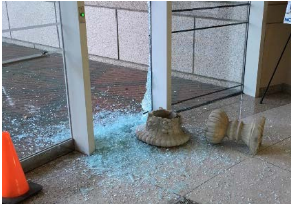
NCDOR Raleigh Headquarters, 4/3/17
