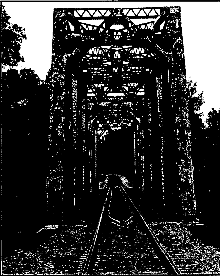
This bridge at Wilsons Mills in Johnston County was constructed in 1927. It has overhead railcar clearance restrictions and is scheduled for rebuild or replacement in 2005-6. (Photo Oct. 2004)
