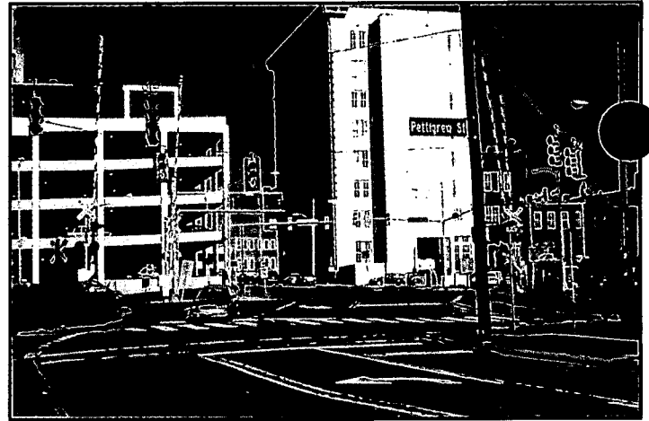
The crossing at Blackwell Street in Durham, adjacent to the American Tobacco Project and the Ball Park, was the site of a train-car collision as recently as December 10. With the addition of TTA trains, there will be freight, Amtrak and commuter rail at this crossing, along with significant pedestrian traffic. As cities and towns have more sidewalk improvement funds available for their use, sidewalks across the NCRR tracks present a growing safety, liability, and maintenance issue. (Photo Nov. 2004)
