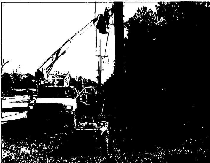
Wynncom installs infrastructure in Haywood County as part of a fiber network.
