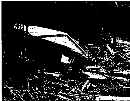
Aftermath of a flood Photo courtesy of Macon County government.
