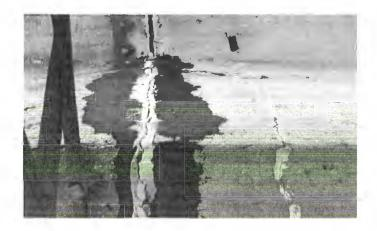
Cracking in stepped slab adjacent to an expansion joint
