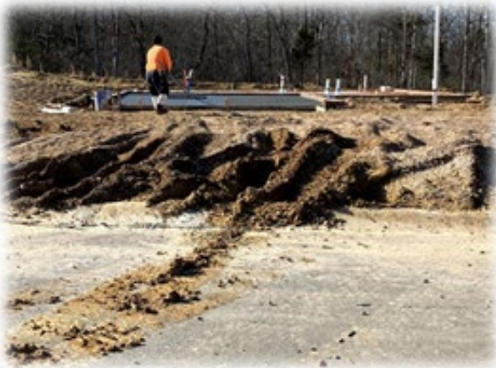
Figure 8 – Poor Construction Entrance
