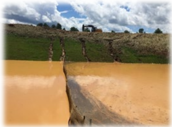
Figure 11 - Rill Erosion on Sediment Basin Slope
