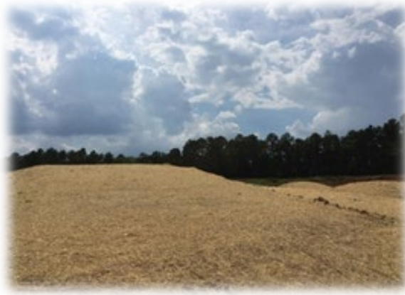
Figure 9 - Good Application of Ground Cover
