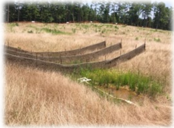
Figure 12 - Good Vegetative Stabilization
