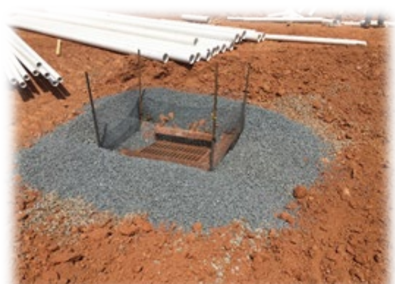
Figure 13 - Good Inlet Protection
