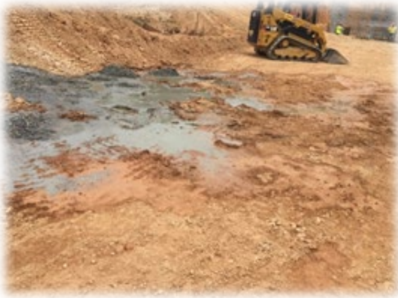
Figure 6 - Unmanaged Concrete Washout
