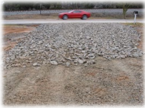
Figure 7 - Good Construction Entrance
