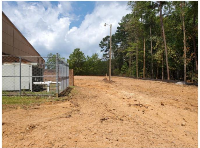
Tree clearing alongside Auditorium
