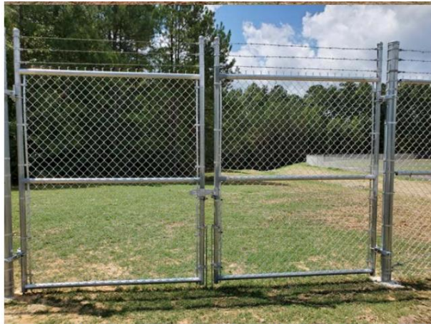
Gate installations. Look good, still need anchor blocks installed
