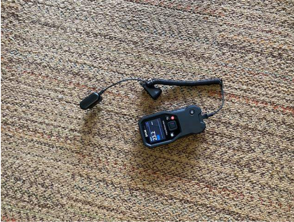
Water intrusion detected under flooring in Entry Hall near lobby.
