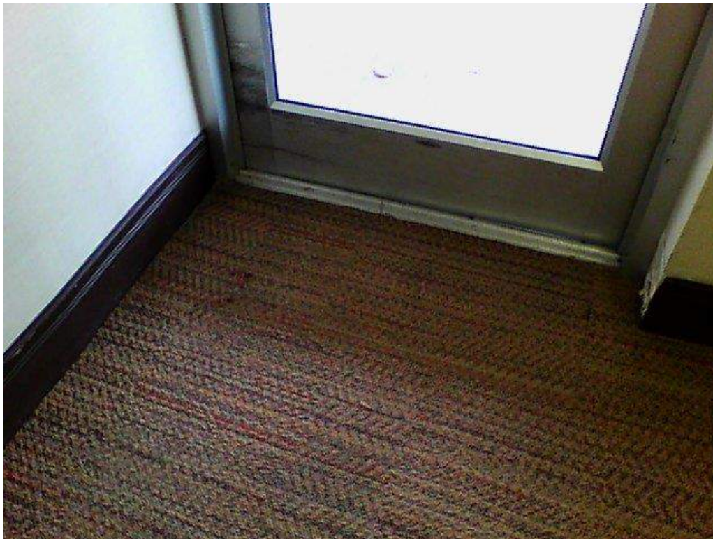
Photograph of image above, located in Entry Hall near Lobby.
