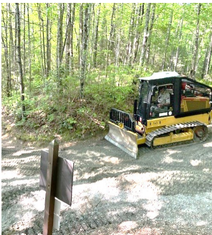
NCFS equipment operator reshapes the surface of the Triple Falls Trail prior to the gravel application.
