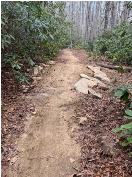
Construction of a turnpike along Grassy Creek Trail eliminates a chronically wet area and improves trail experience for visitors.
